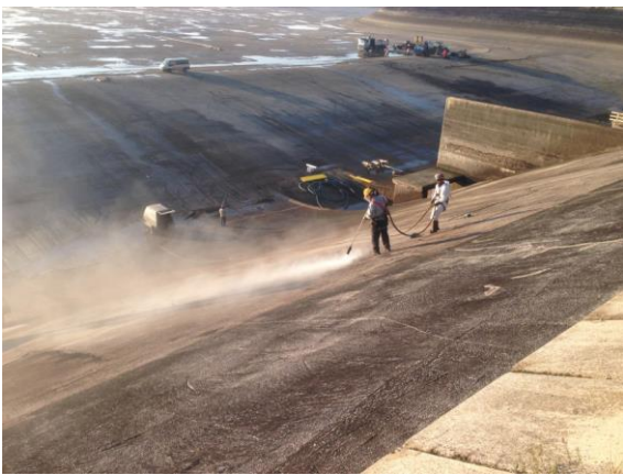
The cleaning operations of the facing
